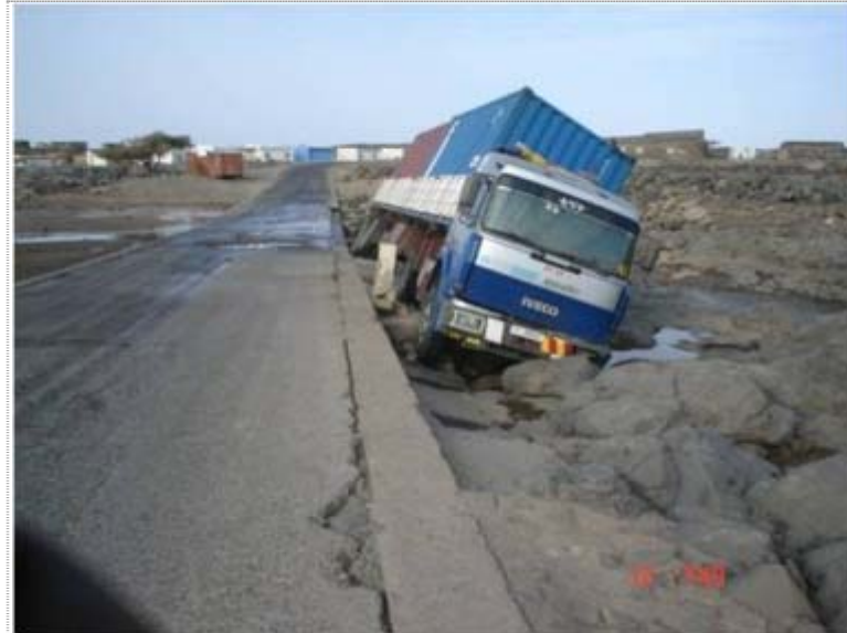
Figure 81. View on the Transafrican 6. Djiboutian Section (Dikhil – MILEAGE POINT 157)
