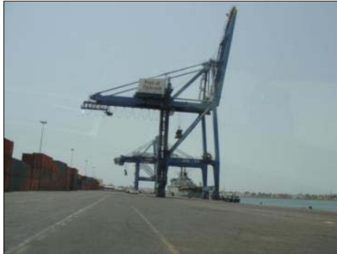
Figure 19. Overview of the new container terminal of Doraleh
