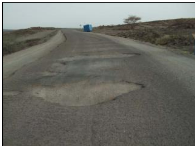
Figure 48. Transafrican 6. Djiboutian Section – General view of Gallafi – Dikhil Section
