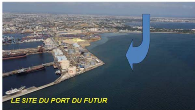
Figure 12. Site of Dakar future port
