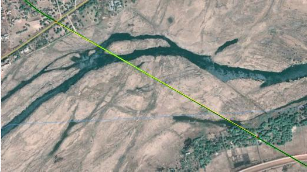
Figure 65. Bridge on Niger river in Bamako (1500 ml)
